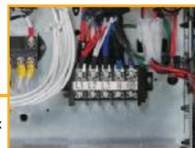
Outdoor unit power supply terminal block
