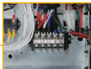
Outdoor unit power supply terminal block
